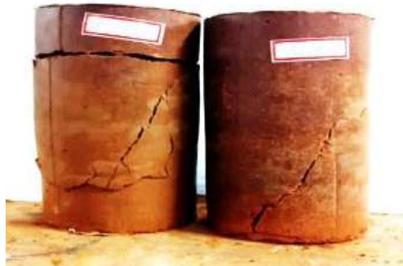
Fig. 10. Failure patterns of specimens reinforced at (A) 2H/4 and (B) H/2 .
