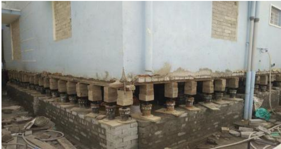
Figure 3: Raising of the House with Jacks
