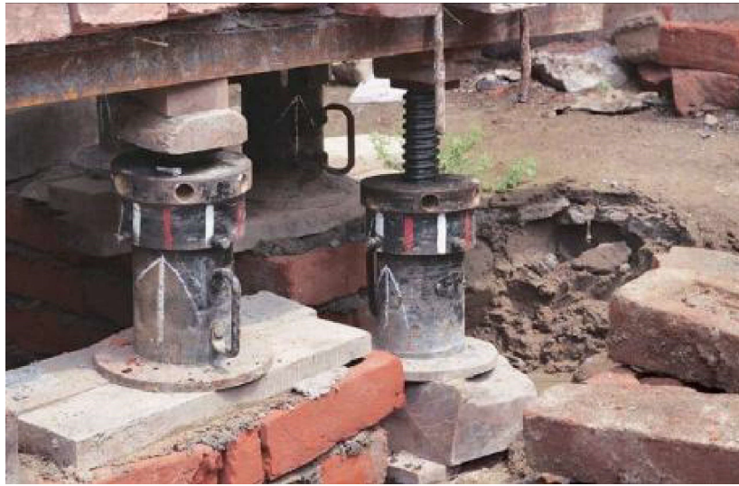
Figure 5: Removal of Jack
