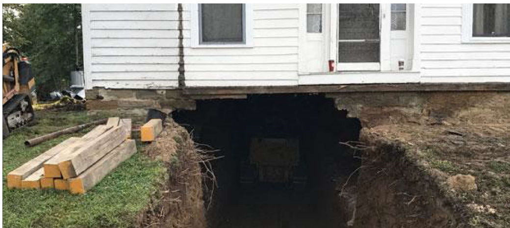
Figure 2: Removal of Soil Under the Foundation
